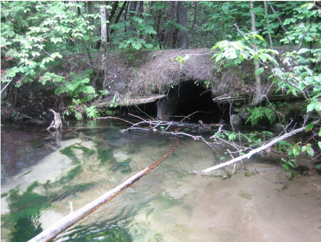
*Culvert inlet with eroding upper bank at Elder Road East on Finch Creek.*
