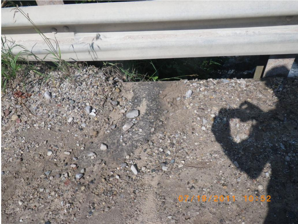
*Sediments pour into the Rapid River from the bridge at Dundas Road.*
