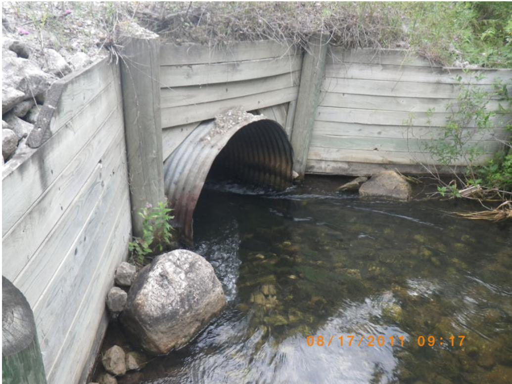
*Sediments fall on to the culvert and into the Little Rapid River at Hill Road.*
