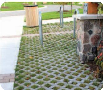
**Porous concrete** is composed of materials that result in voids when it is dry, allowing water to drain through a bed of stone
