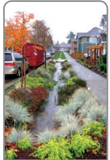
Example of a bioswale in action.
