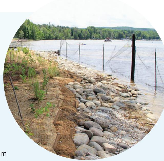
Another option for inland lakes is bioengineering. Bioengineering is a form of erosion control that incorporates biological, ecological, and engineering concepts to produce a living, functioning shoreline system through the use of live and dead plant material, native soils, and structural materials.
