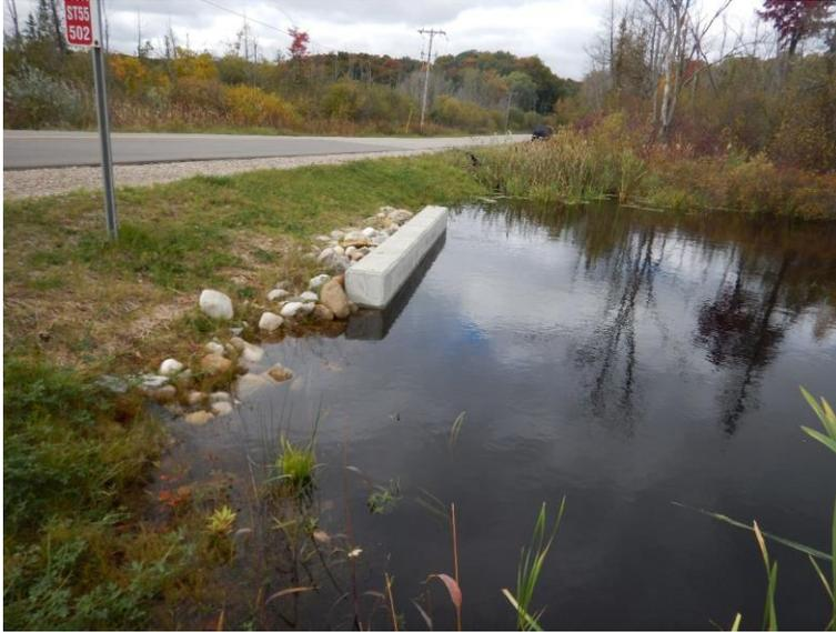
Figure 12. The new concrete box culvert on Fineout Creek/E. Shadow Trail
